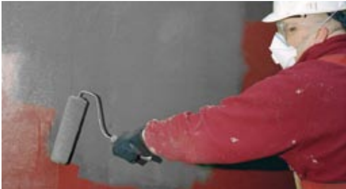
Chemically resistant SikaGard coating being applied
